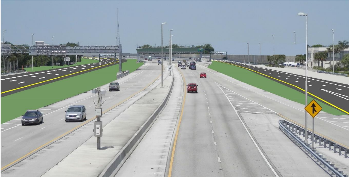
View of the Sawgrass Expressway, from Florida's Turnpike, after the tollbooths are removed and the project is completed.
