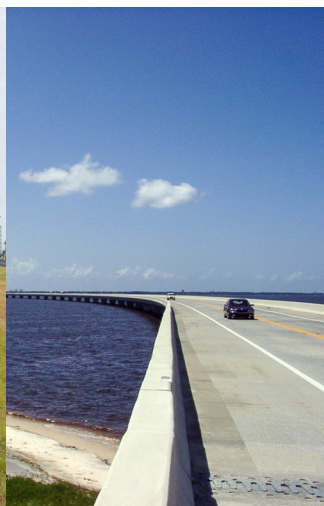
Garcon Point Bridge
