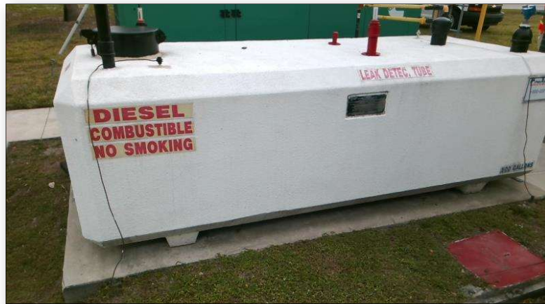
Figure 21 Fuel tank Missing Tie Down Straps
