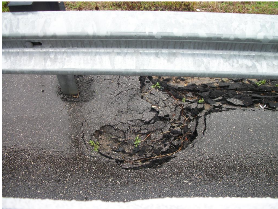
Undesired Guardrail Asphalt Condition – Deterioration
