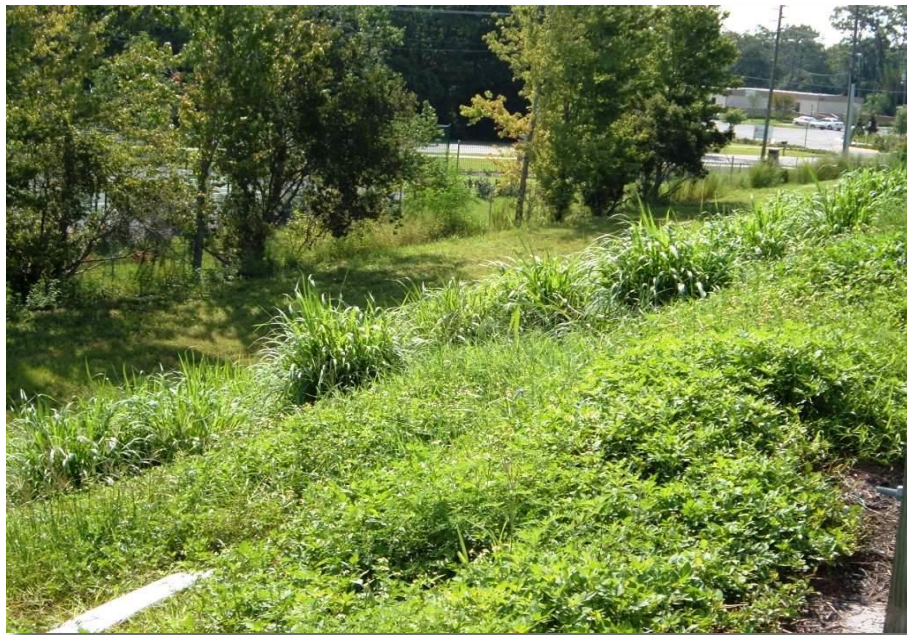
Undesired Soil, Shoulder and Front Slope Condition – Vegetation
