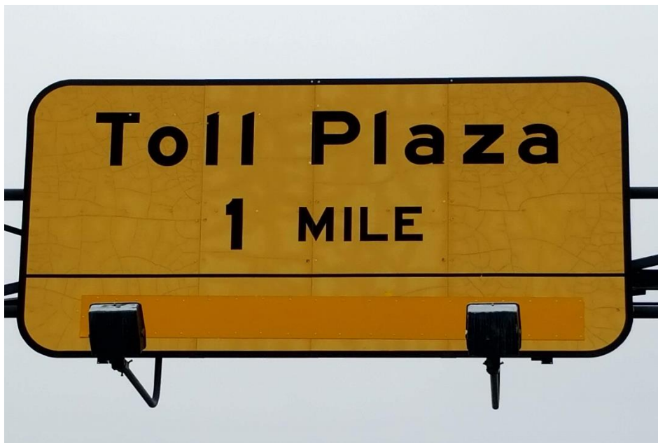
Undesired Sign Reflectivity Condition – Material Cracked and Faded
