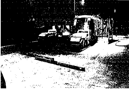
Checking cross slope of subgrade following milling of existing limerock base
