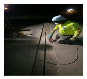
Bridge joint prior to the installation of the polymer nosing system
