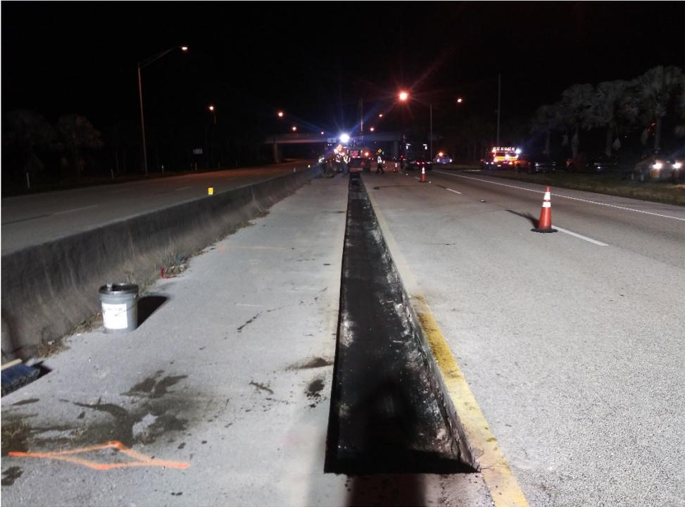
2) H-20 Loaded Traffic Grate for Drainage Structure S-1
