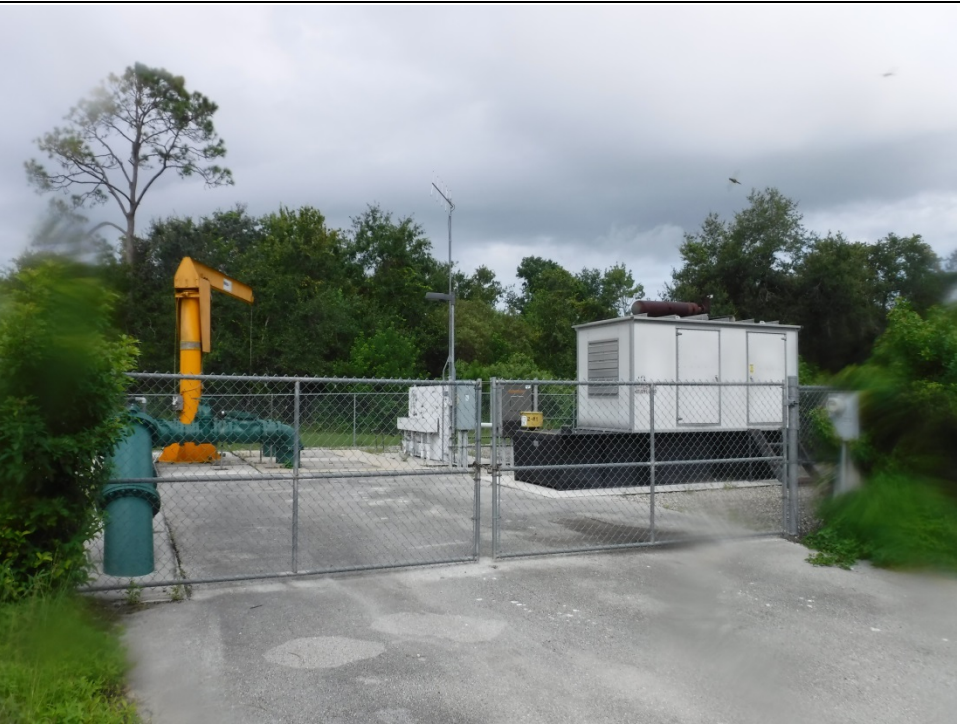
Looking west toward the existing lift station. The emergency generator and belly tank are on the right.
