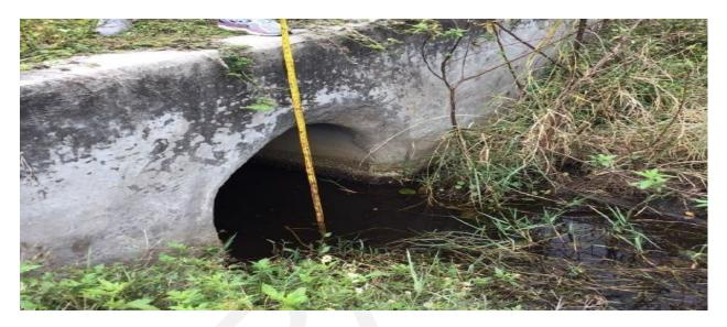
Figure 2-4: CD-3 (36-inch Reinforced Concrete Pipe) at MP 240.7 (Photo taken 1/23/2019)
