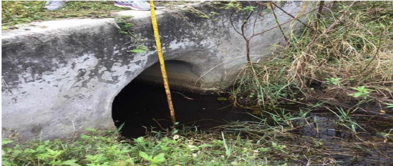
Figure 2-4: CD-3 (36-inch Reinforced Concrete Pipe) at MP 240.7 (Photo taken 1/23/2019)
