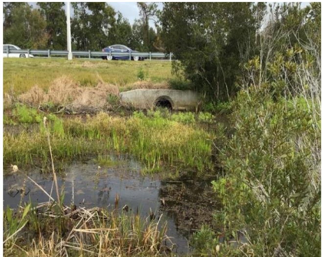
Figure 2-3: CD 2 (42-inch steel pipe) at MP 239.7 (Photo taken 1/23/2019)
