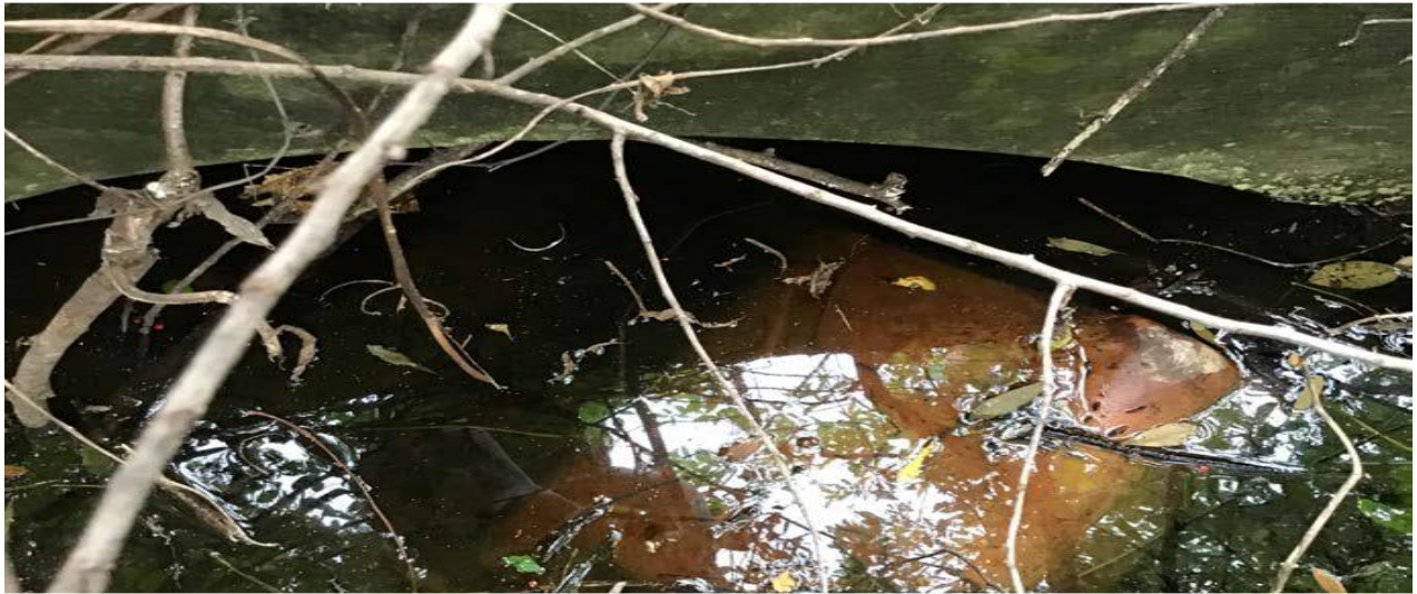
Figure 2-5: CD-5 (Double 36-inch RCP) at MP 242 (Photo taken 1/23/2019)
