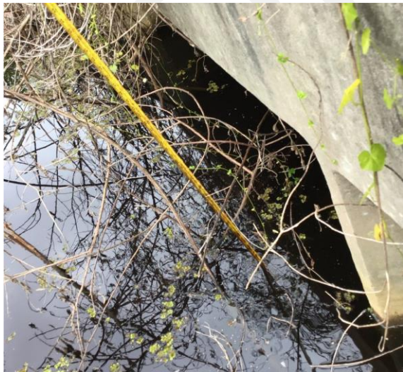
Figure 2-2: CD-1 (Double 7-foot by 4-foot Concrete Box Culvert) at MP 239.5 (Photo taken 1/23/2019)
