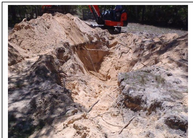
Photo 6. A photo of a fully excavated burrow and end chamber in advance of backfilling / regrading.
