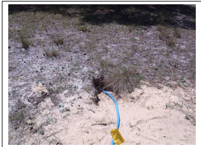
Photo 4. A photo of pvc pipe chasers placed into burrows in advance of excavation in accordance with FFWCC guidelines.
