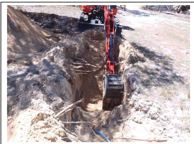
Photo 5. A photo of back-hoe in process of excavating burrows on-site.
