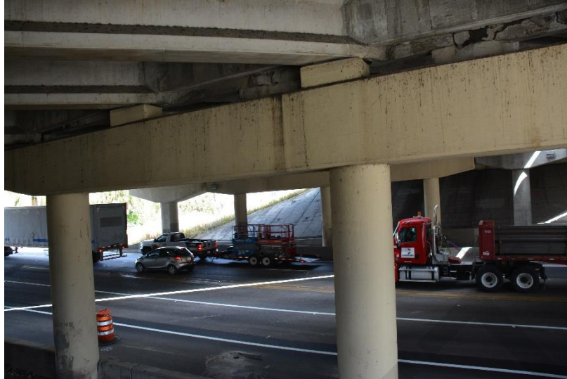
Representative Bridge Structure
