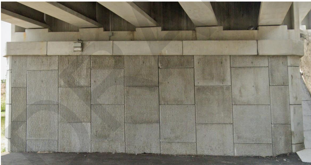
Figure 6 Sample Wall Aesthetics – Uncoated Vertical Fractured Fin Retaining Wall Texture (SR 91 Loop Ramps)
