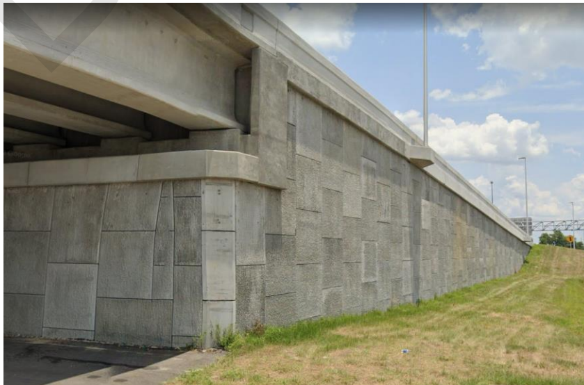
Figure 2 Uncoated Concrete Surfaces and Retaining Walls
