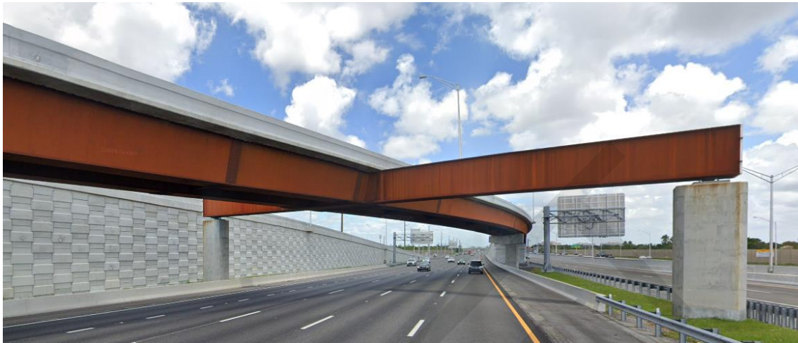
Figure 1 Uncoated Weathering Steel Bridge, Uncoated Concrete Surfaces and Retaining Walls (I-75 SB Express Lanes Off-Ramp over I-75 SB General Purpose Lanes)
