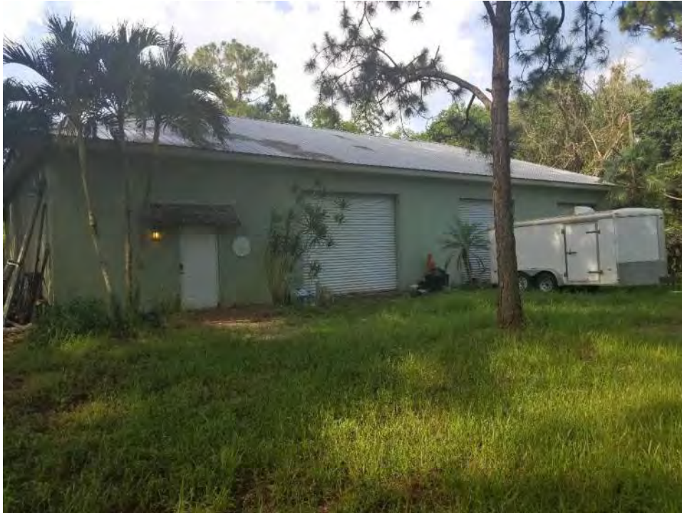
SMF 39-2: storage building (unoccupied, locked) and storage trailer associated with abandoned tree farm located in eastern area
