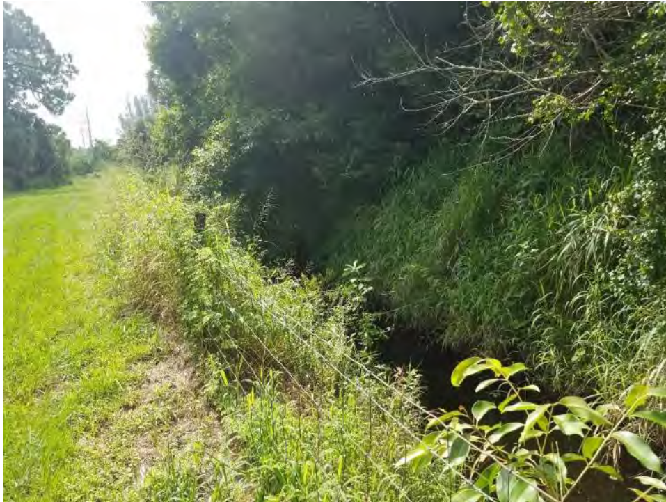
SMF 39-1 access easement: east end of easement looking east
