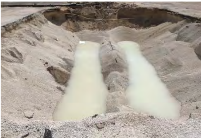
Base of Excavation After USTs Removal Looking West
