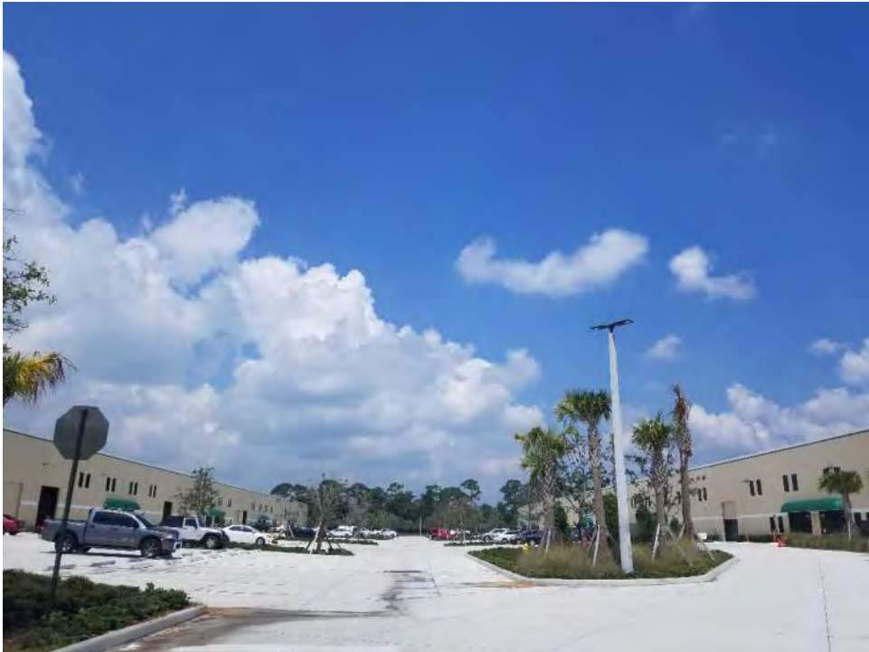
SMF 41-2 and SMF 41-3B: east-central area looking west
