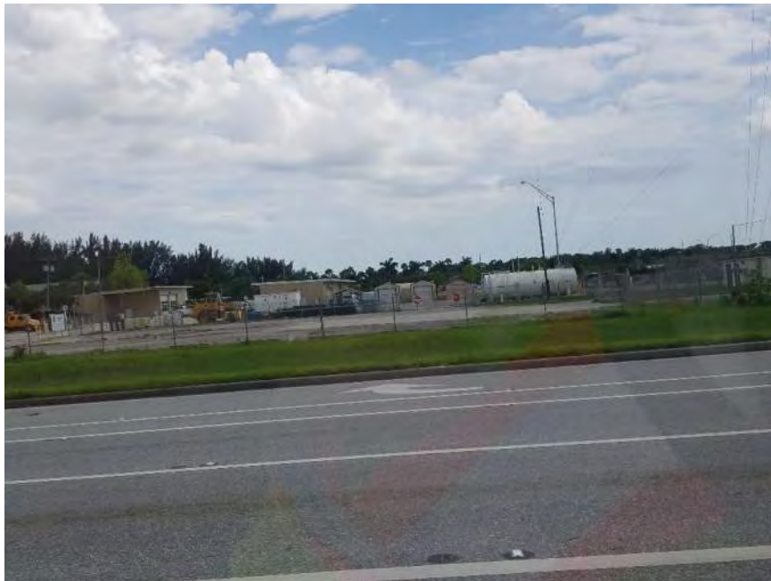
Site 23 - FDOT Turnpike MM 133 Martin County/Stuart Maintenance Yard North side looking south
