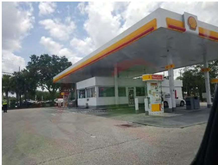
Site 66 - Port St. Lucie Shell/ Former Chevron Southeast looking northwest
