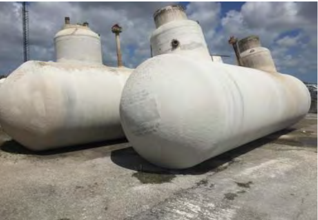
USTs After Removal From Excavation
