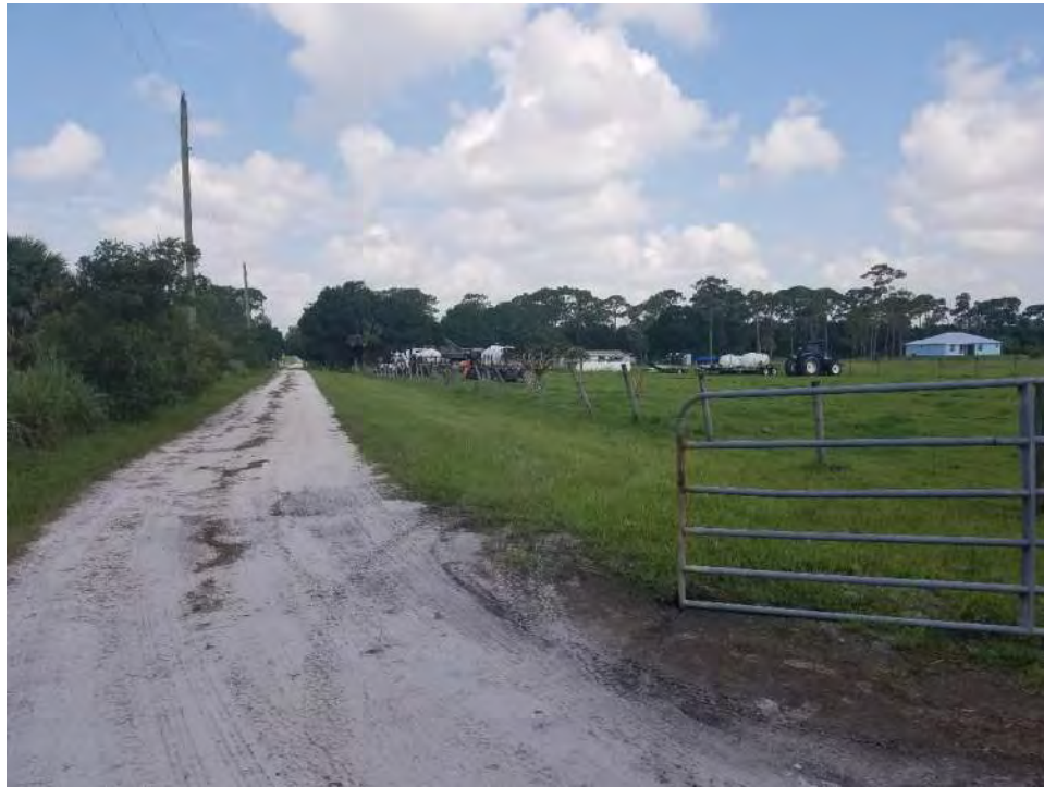
SMF 39-1 access easement: west end of easement looking west
