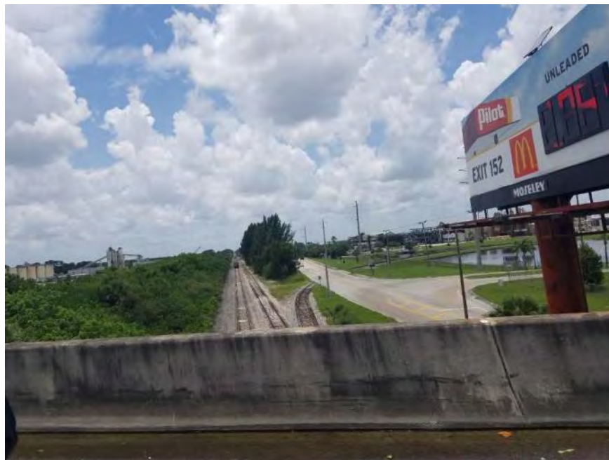
Site 91 - Railroad Track Florida's Turnpike bridge over railroad tracks looking west
