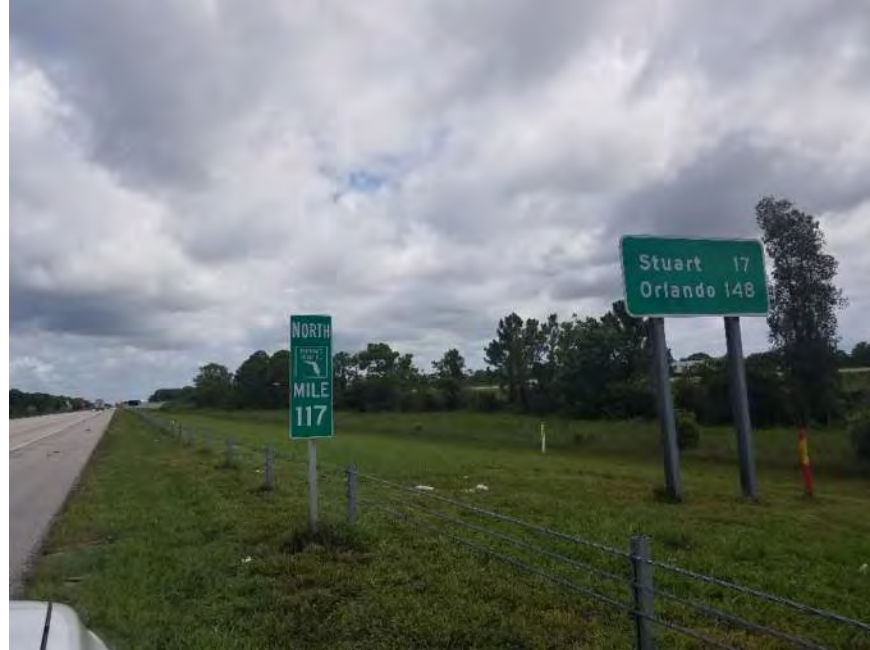
South end of project looking north
