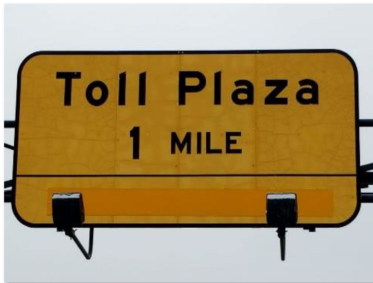
Undesired Sign Reflectivity Condition – Material Cracked and Faded
