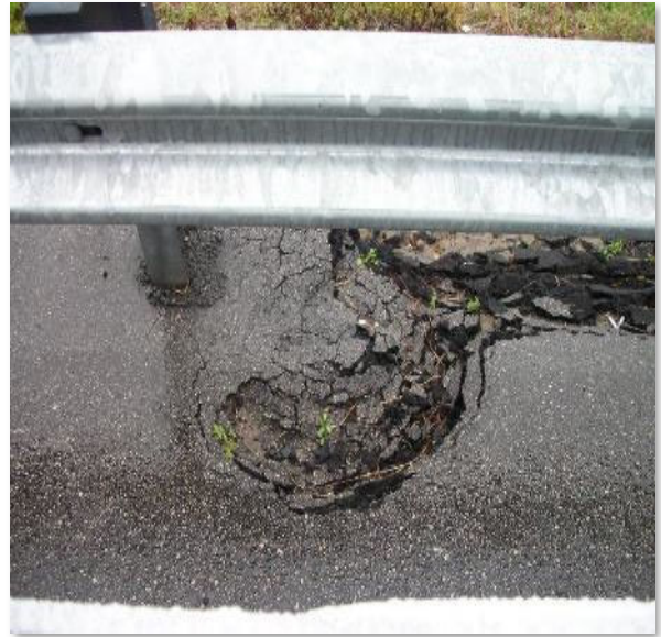
Undesired Guardrail Asphalt Condition – Deterioration
