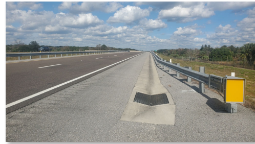
Figure 11: Typical Paved Shoulder / Shoulder Gutter
