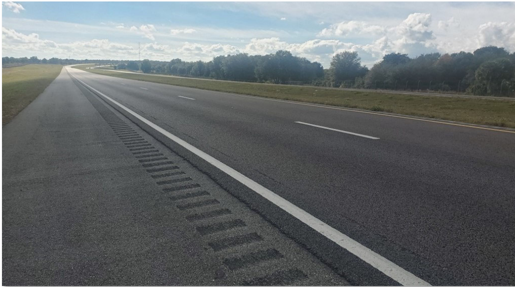
Figure 9: Typical Paved and Soil Shoulder Section
