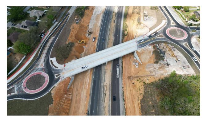
This work is part of the widening of Florida's Turnpike/SR 91 from Clermont/SR 50 to Minneola/Hancock Road. The bridge reconstruction was necessary to accommodate the Florida's Turnpike widening, from four to eight lanes.
