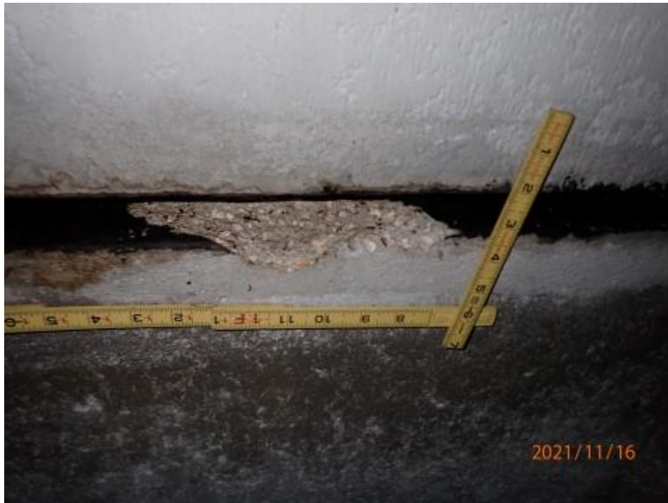
Element 241: Photo 9 - Typical Edge Spall at the Joints
