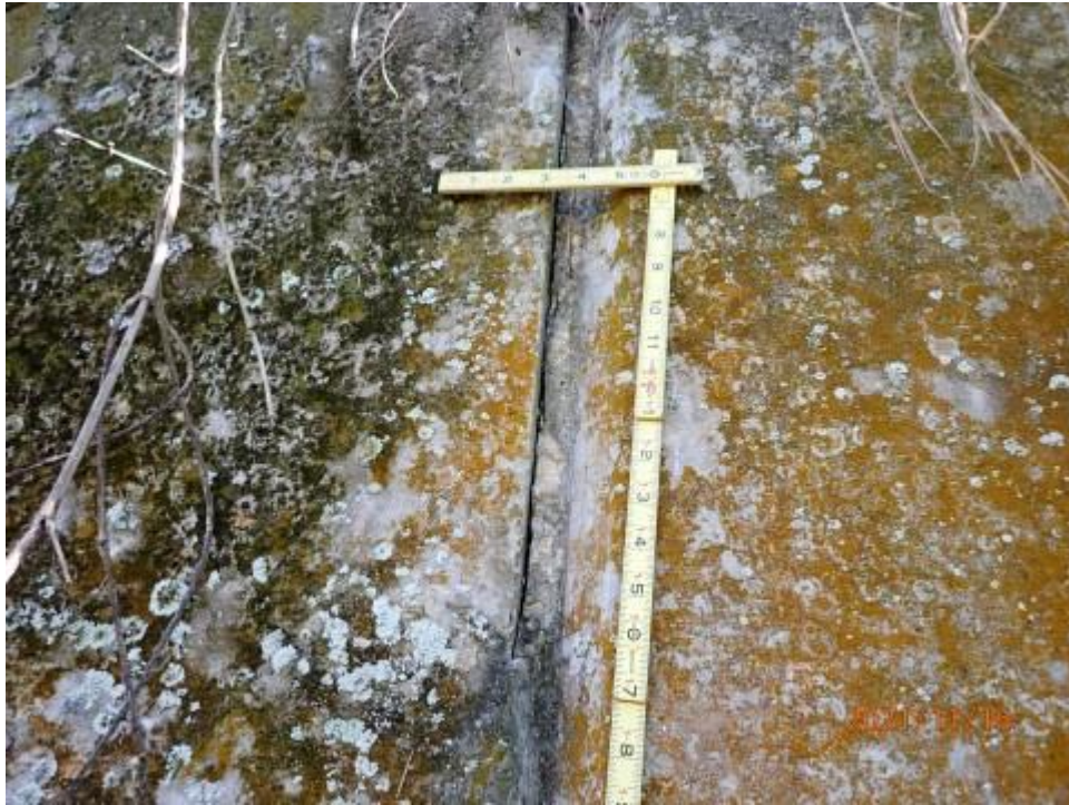
Element 8475: Photo 7 - Spall in the Southwest Headwall/Wing Wall Joint
