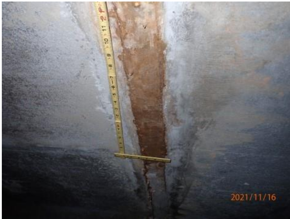
Element 241: Photo 10 - Typical Crack in Grouted Joint with Efflorescence, Corrosion Bleedout and Water Leakage
