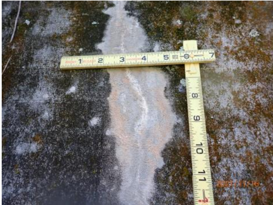
Element 241: Photo 11 - Typical Vertical Crack with Efflorescence in Headwall
