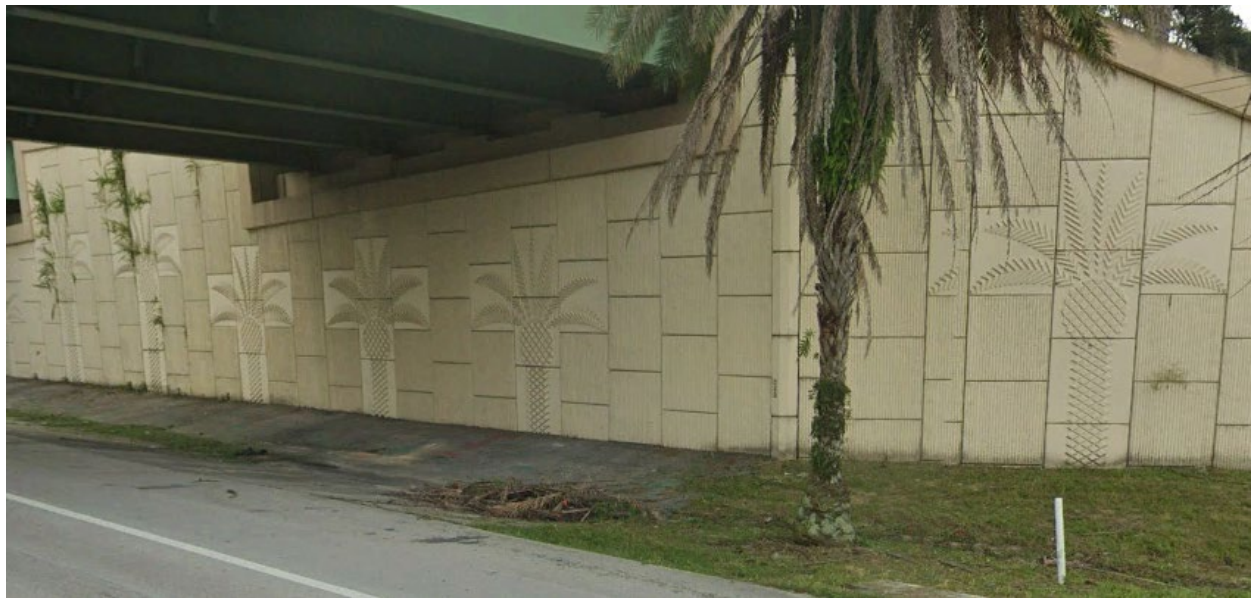
Figure 2-29: MSE Walls at the US 192 Interchange
