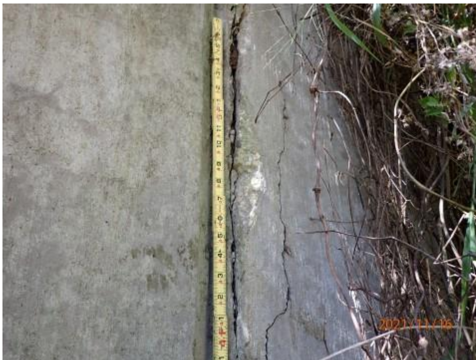
Element 8475: Photo 6 - Spall/Impending Spall in the Northeast Wing Wall/Headwall Interface
