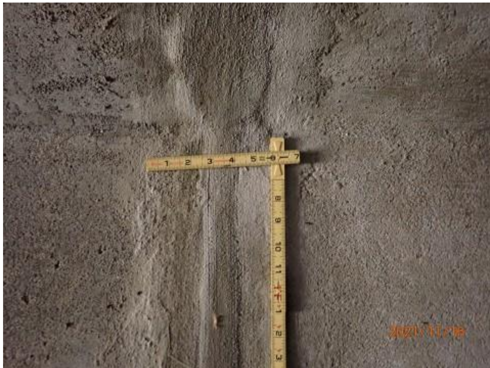
Element 241: Photo 12 - Typical Grout Coat in Joint Full Circumference
