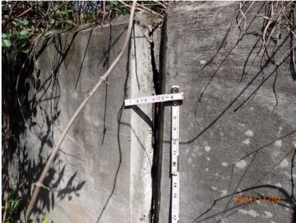
Element 8475: Photo 7 - Vertical Crack in the Northwest Headwall/Wing Wall Joint
