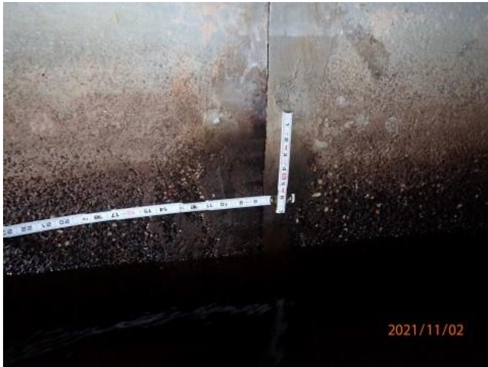
Element 241: Photo 9 - Typical Vertical Crack with Corrosion Bleed-Out in the Construction Joint
