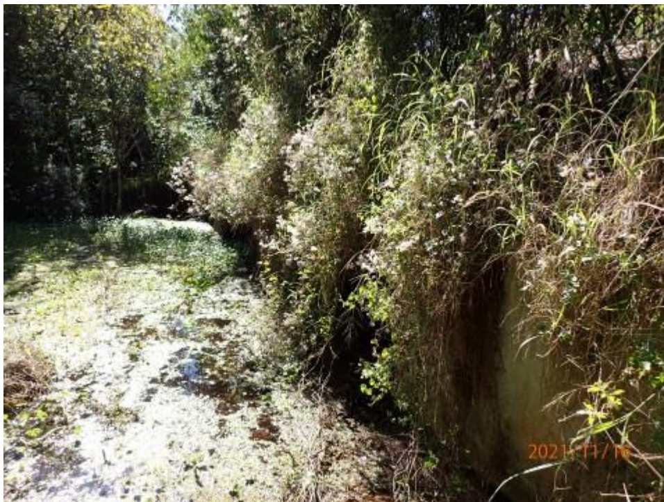
Element 8290: Photo 3 - Typical Heavy Accumulation of Vegetation at Ends of Cell
