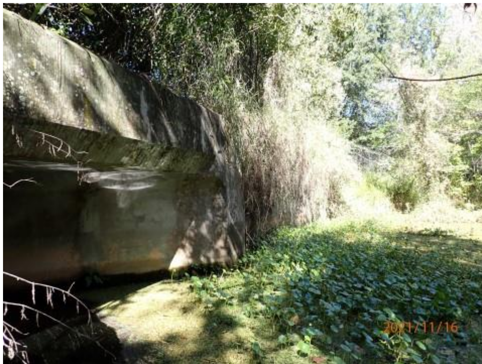
Element 241: Photo 13 - Typical Headwall Overgrown with Vegetation
