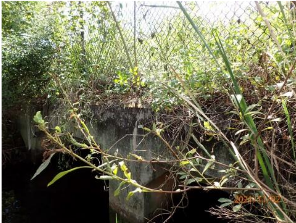
Element 241: Photo 11 - Typical Headwall Overgrown with Vegetation
