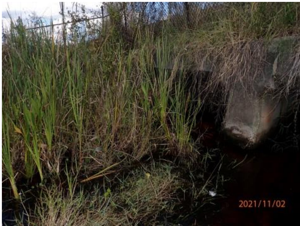
Element 8290: Photo 3 - Vegetation Growth Restricting Flow in Cell 2
