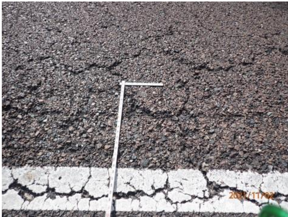
Element 241: Photo 10 - Typical Crack in the the Travel Lane
