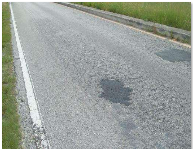
Undesired Travel Lane / Ramp Condition – Deterioration
