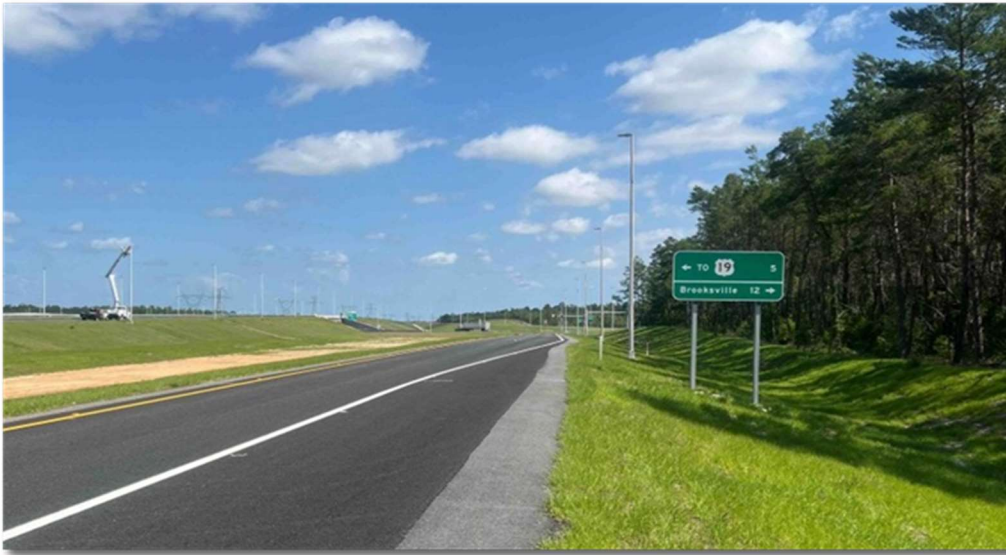
Figure 9: Typical Paved and Soil Shoulder Section
