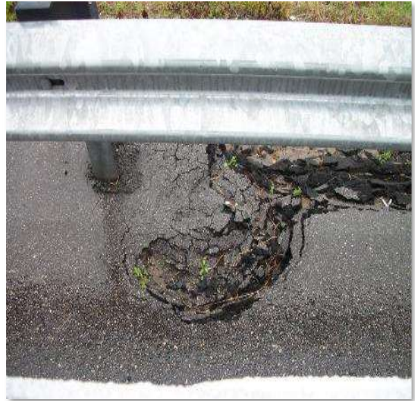
Undesired Guardrail Asphalt Condition – Deterioration
