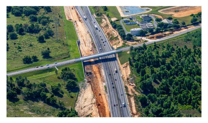
This work is part of the widening of Florida's Turnpike/SR 91 from Minneola/Hancock Road to north of O'Brien Road. The bridge reconstruction was necessary to accommodate the Florida's Turnpike widening, from four to eight lanes.
