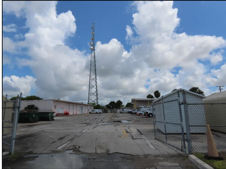
Figure 4-8: FDOT Southern Regional Office maintenance yard, with the two contributing concrete block maintenance buildings visible, facing north (Janus Research 2023)
