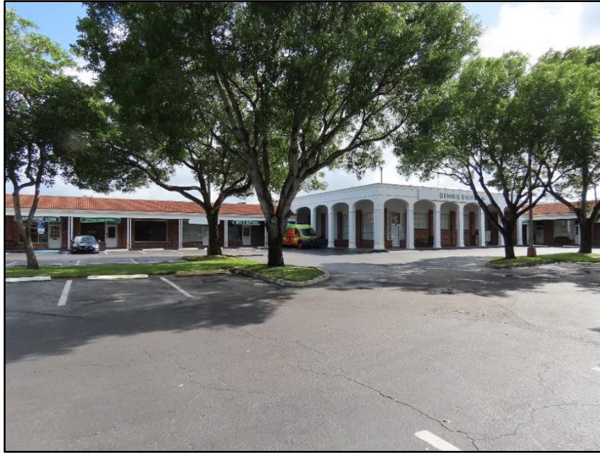
Figure 4-3: West wing and arcade of Plantation Village Shopping Center (8BD8428), facing northeast (Janus Research 2023)
