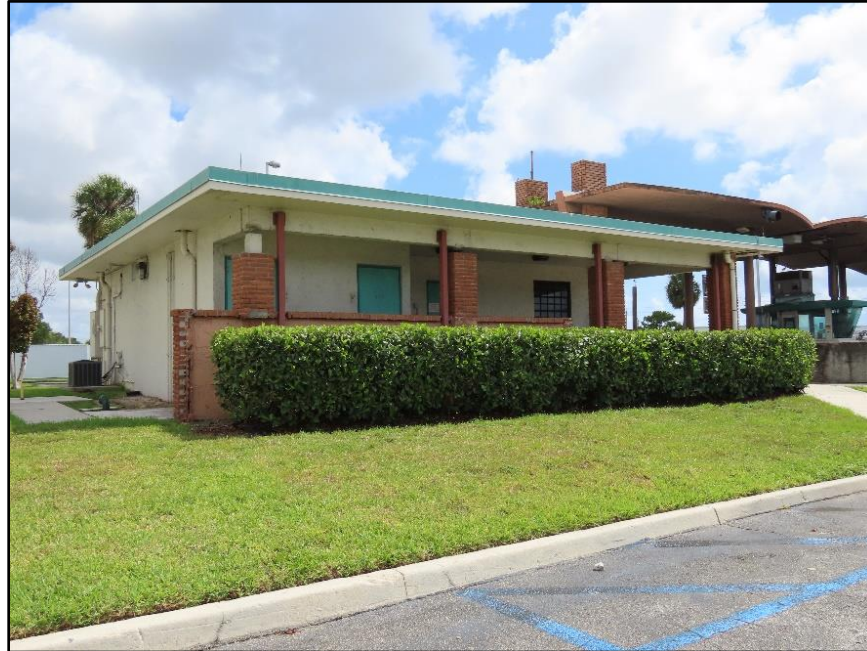
Figure 4-6: FDOT Turnpike Southern Regional Office building, a contributing resource, facing northeast (Janus Research 2023)
