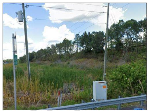
Figure 2-17: Existing Load Center and Service Point on SR 54
