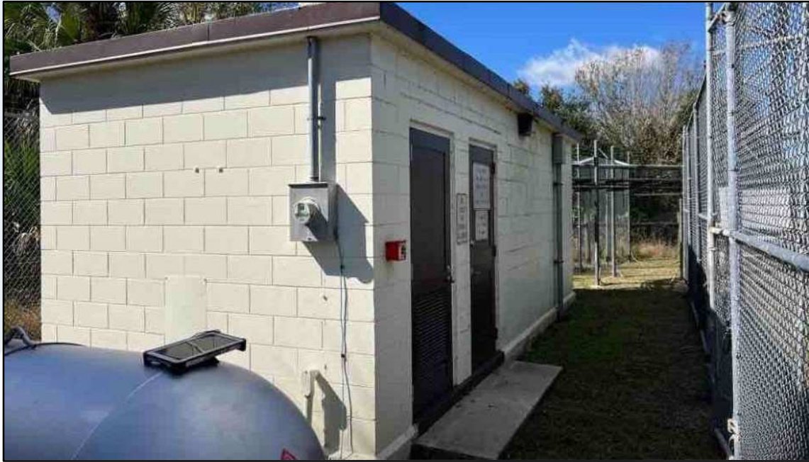
Figure 4: Delray Communications Building Exterior
