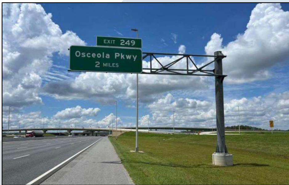
Figure 8: Overhead Sign Structure
