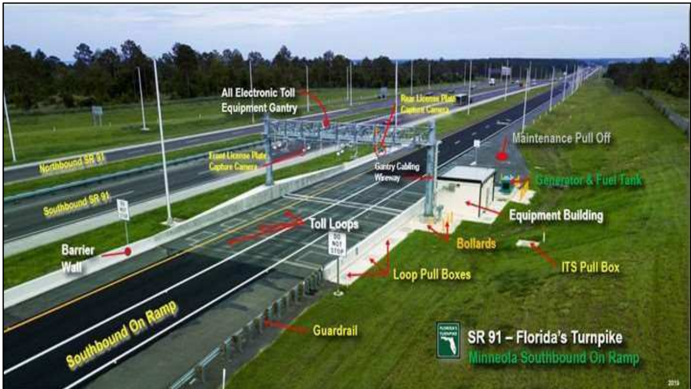
Figure 3: AET Toll Collection Point Elements
