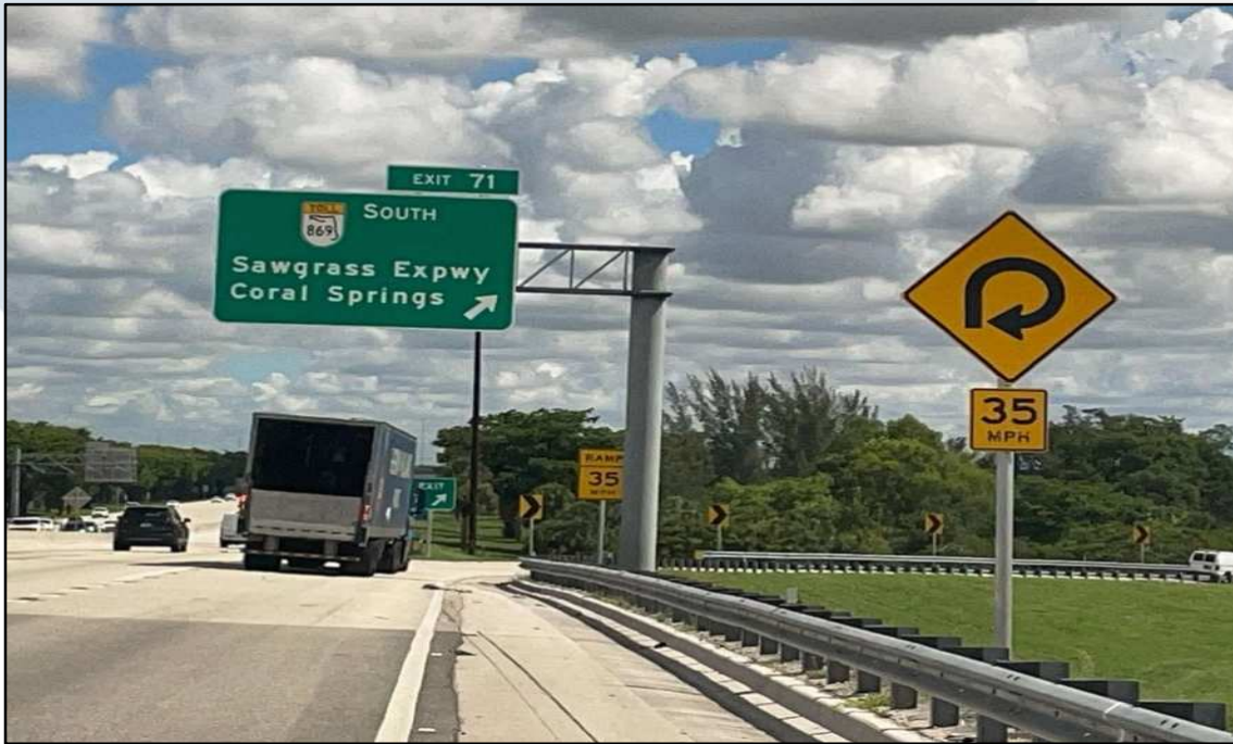
Figure 16: Typical Overhead Sign Structure
