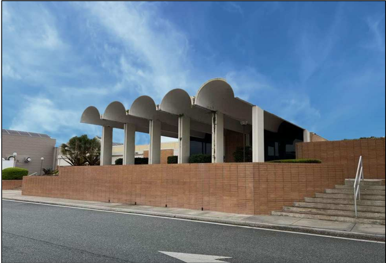
Figure 6: Turkey Lake Regional Tolls Building - SR 91
