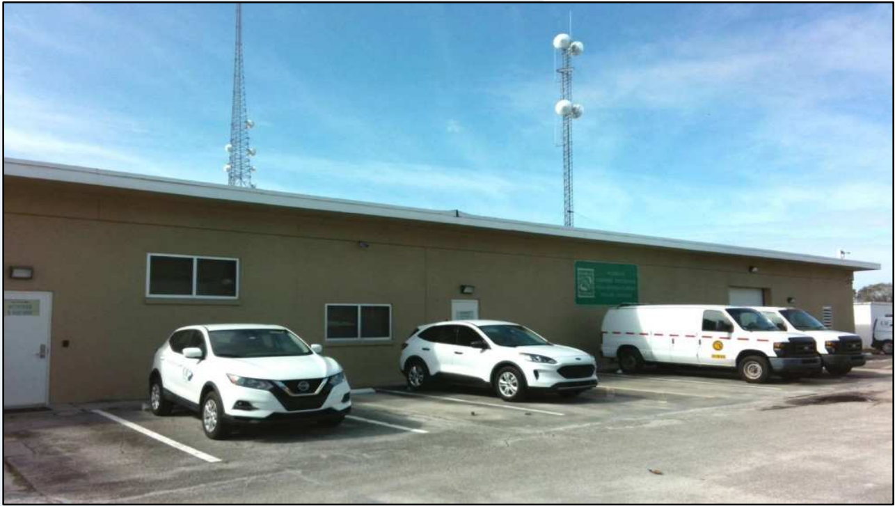
Figure 7: Stuart Maintenance Shop - SR 91
