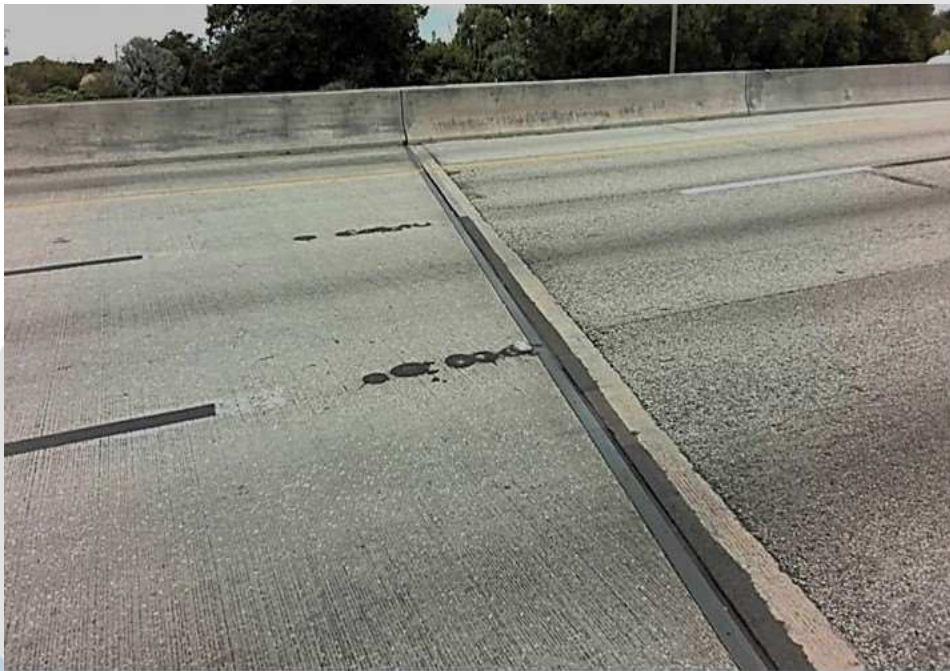
Figure 6: Desired Joint Condition
