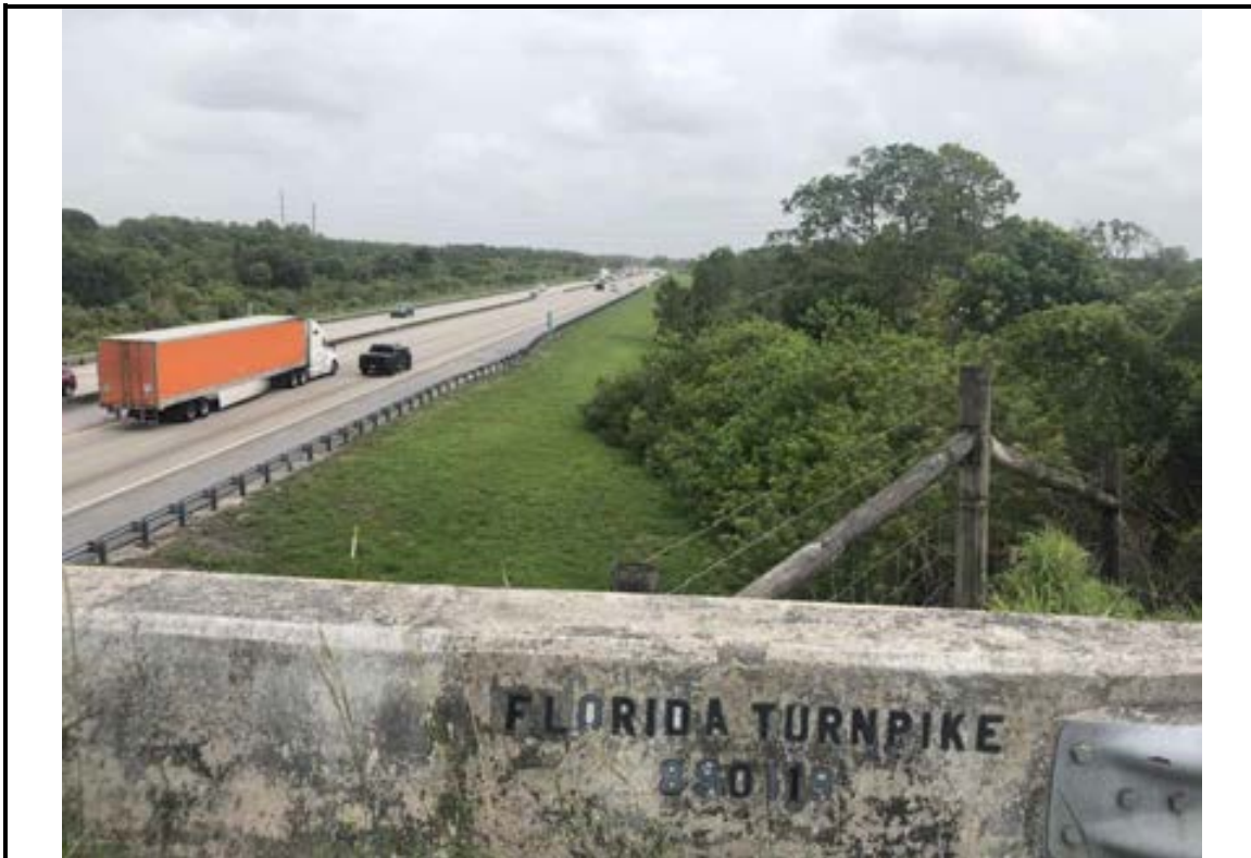
Photo 9 Bridge 890119 over SR91, looking north
