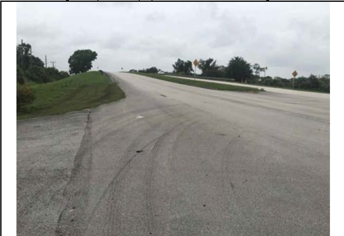
Photo 8 Looking west at Bridge Road over SR91
