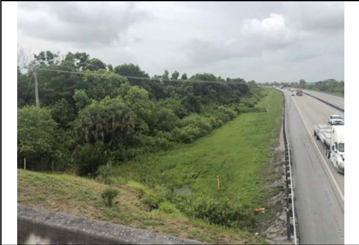
Photo #1 Looking north of Bridge Rd at wooded proposed R/W along southbound side of SR91
