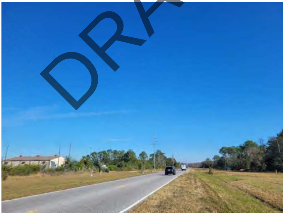
Looking east along Osceola Polk Line Road from northernmost limit
