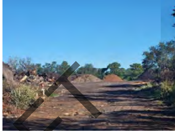
Piles of Processed Material
