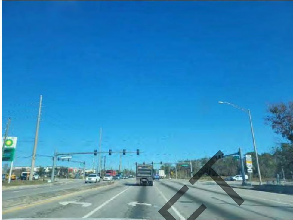
Looking north towards the US 17/92 and Ronald Reagan Parkway Intersection
