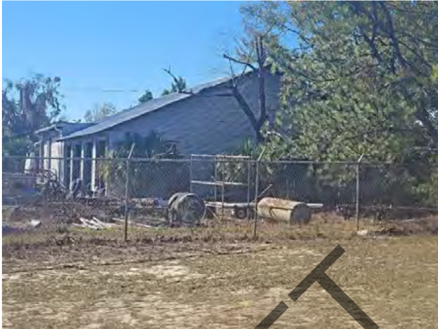
Map ID 6: Tanks observed on site, no secondary containment visible
