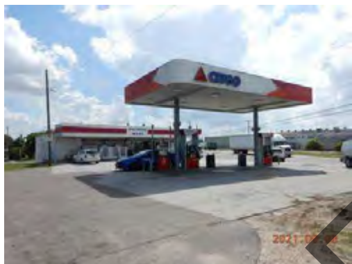
2021-09-08 General Site Photo
