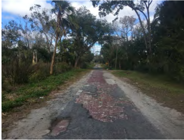
Figure 3.1.4: Old Tampa Highway Trail
